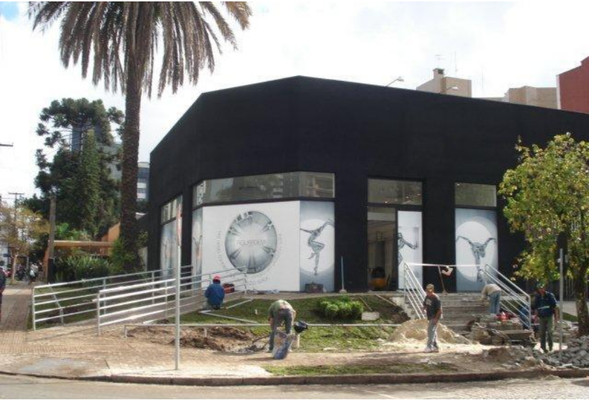
Construction of the soon the be opened shop in Curitiba, Brazil.
